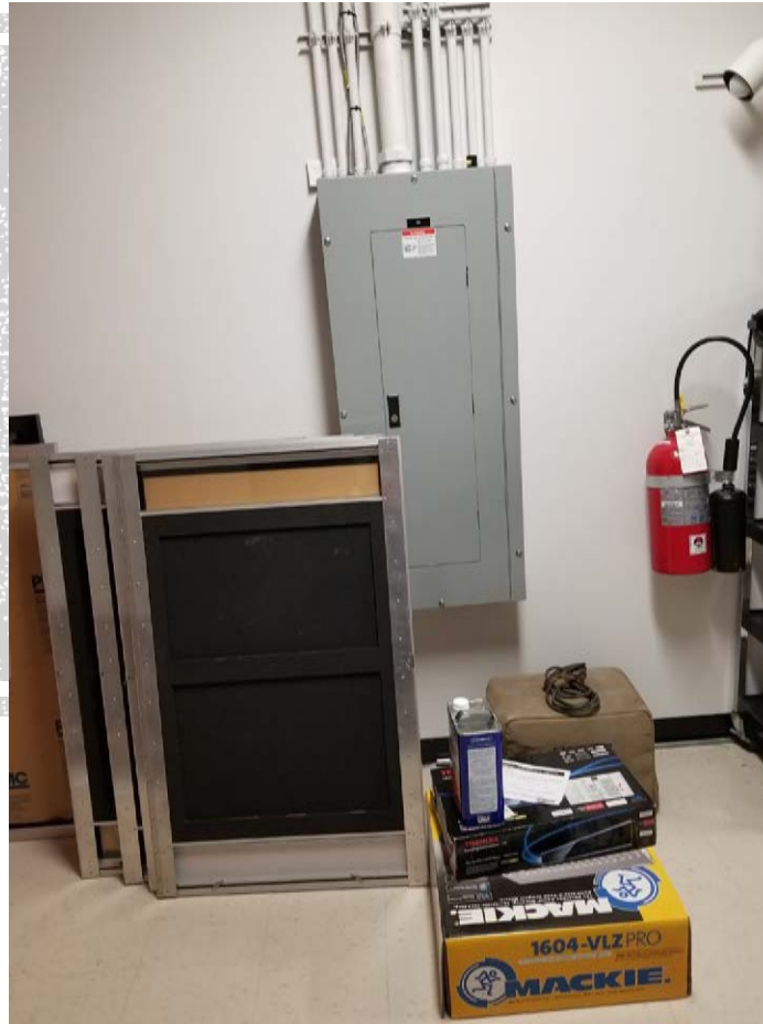
Blocking Electrical Panels
