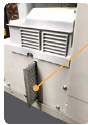
Makeup air passes through Merv 8 filter
